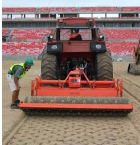
Machine Blending ATS into Top Layer
